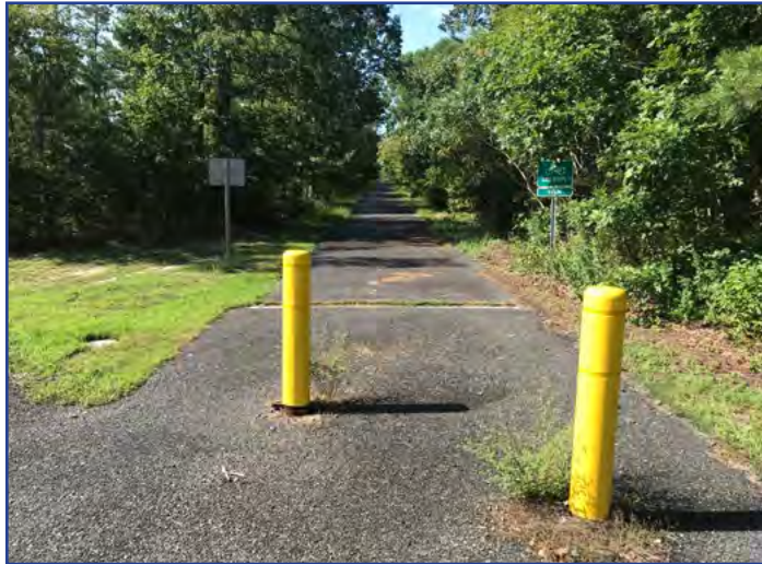
Entrance to the Airport Spur Bicycle Path
